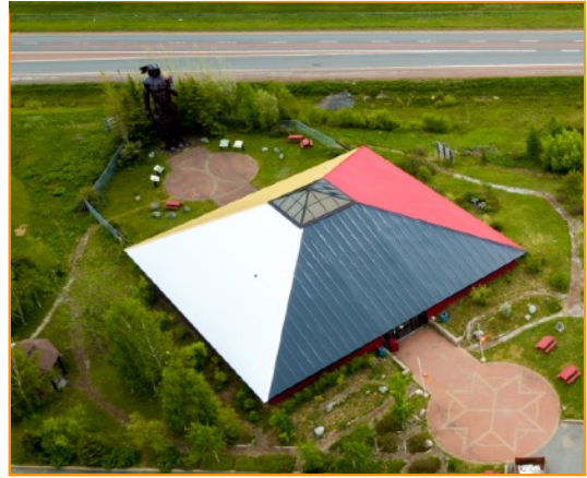
"Millbrook Cultural and Heritage Centre new roof painted in four colours"
